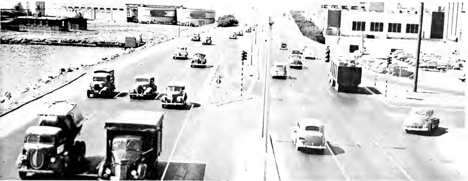
Traffic Signal Control is amplified by channelization islands and separate lanes for turning vehicles
